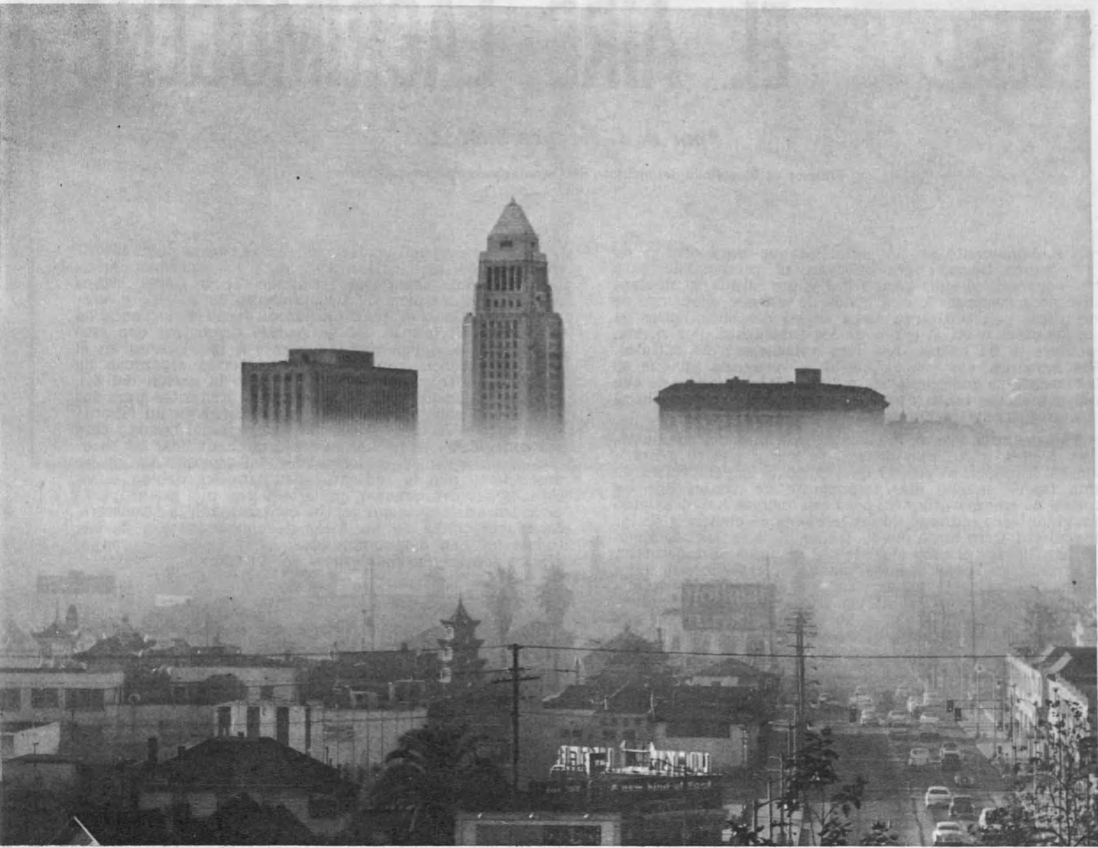
Air Pollution Control District, Los Angeles
